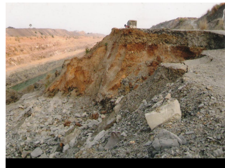
(Bank sliding at RD 34.10 to 34.20 km of LBC)
