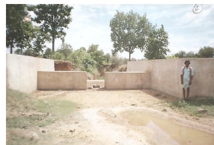
Check dam of Banamouli without sluice gate
