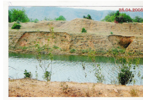
(Damaged canal embankment at RD 8.00 km to 8.04 km due to absence of CC lining)
